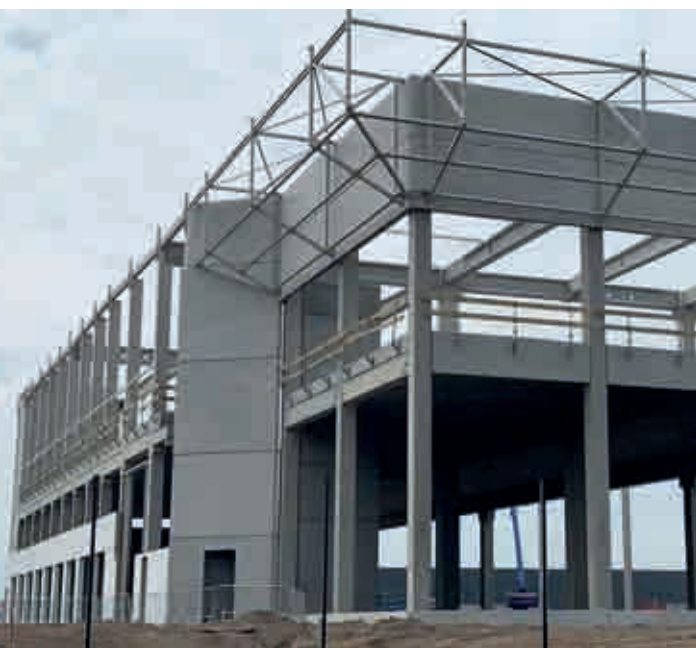
AT GHENT LOGISTIC CAMPUS FOURTEEN UNITS WILL BE CONSTRUCTED.
