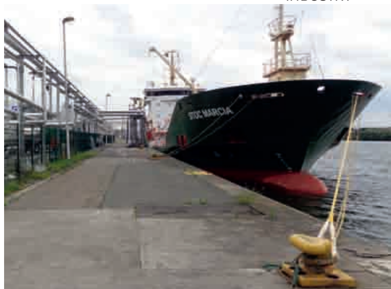
LIQUID BY-PRODUCTS SUCH AS COAL TAR, NAPHTHALENE, AND CRUDE BENZENE ARE SHIPPED FROM ALL OVER THE WORLD TO THE ZELZATE FACILITY.
