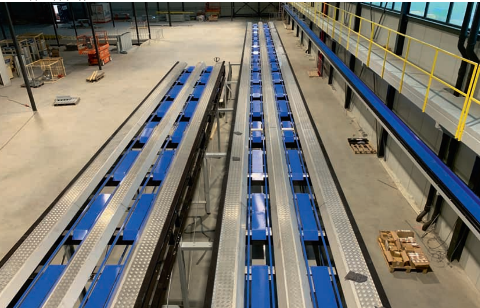
THE PROCESS IS FULLY ELECTRIFIED AND READY TO USE GREEN ENERGY.
