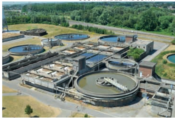
THE WASTEWATER TREATMENT SYSTEM HAS A CAPACITY OF 23,000M 3 A DAY.
