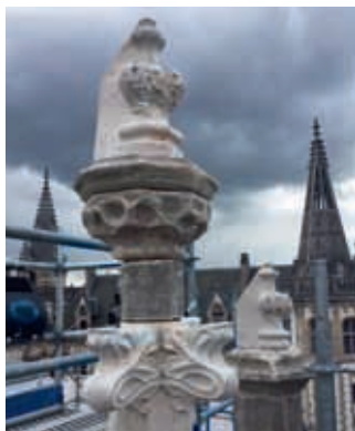
ERODED STONES WERE REPLACED BY ORIGINAL BALEGEM STONES.
