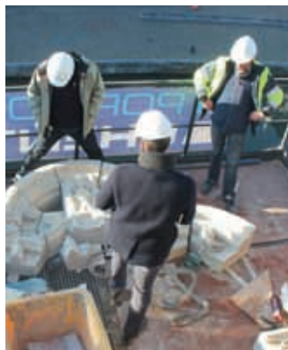
ERODED STONES WERE REPLACED BY ORIGINAL BALEGEM STONES.
