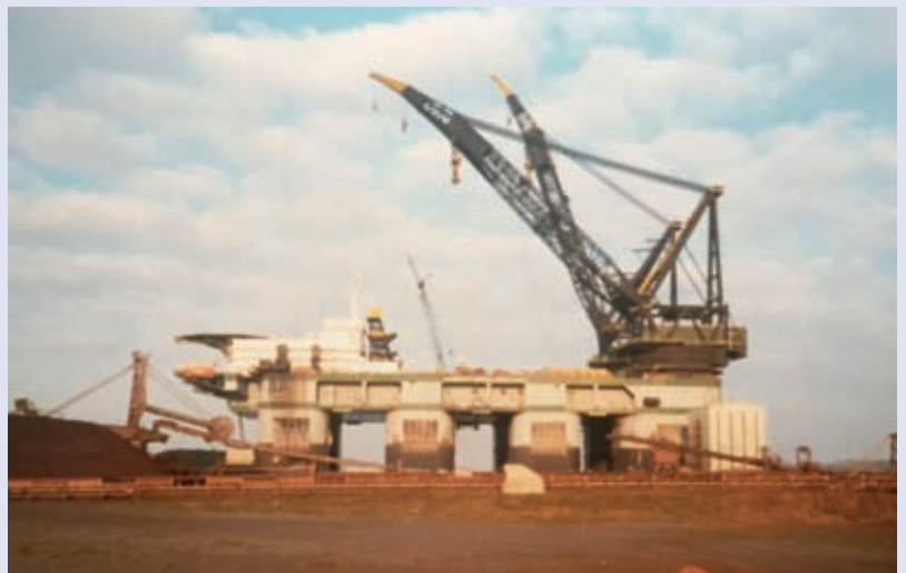
THE THIALF IS A SEMI-SUBMERSIBLE CRANE VESSEL THAT WAS BUILT IN 1985. THE TWO CRANES HAVE A LIFTING CAPACITY OF 14,200 TONNES, MAKING THE THIALF THE LARGEST CRANE SHIP IN THE WORLD.
