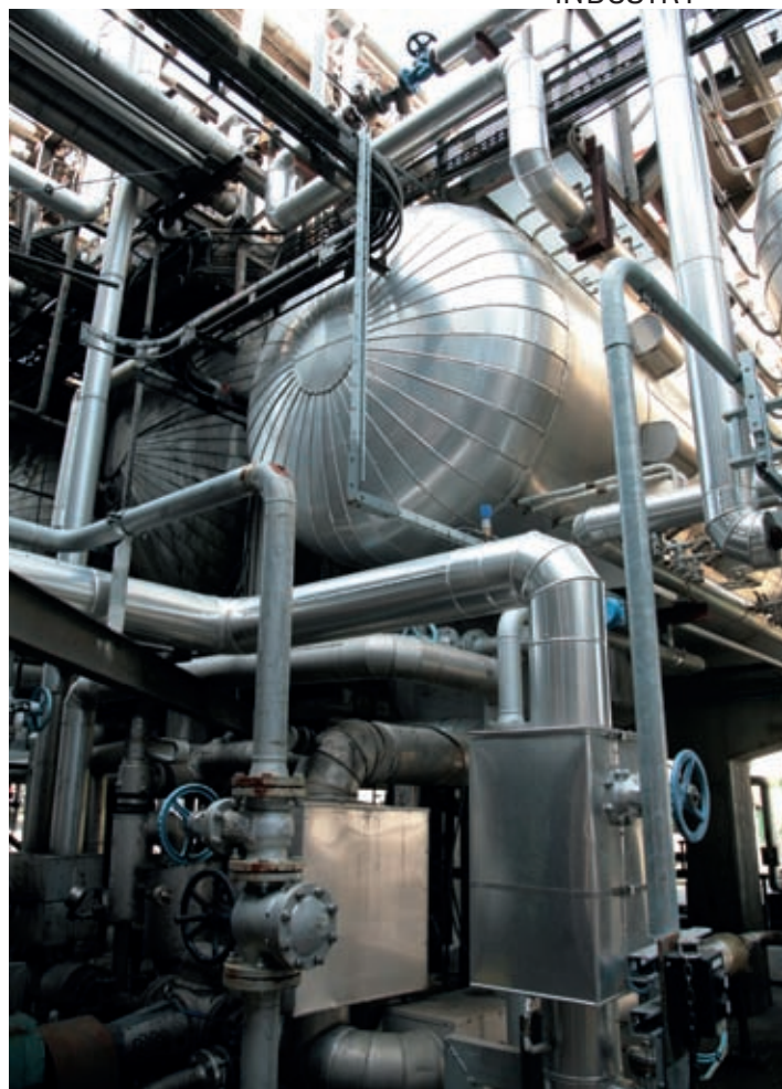
A REACTOR WITH DEDICATED EQUIPMENT, HORIZONTALLY POSITIONED. THIS TYPE OF INSTALLATION IS USED TO PERFORM CHEMICAL REACTIONS.
