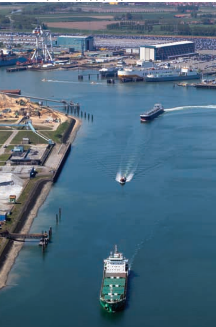
NORTH SEAPORT HAS A DRAFT OF 17M AND IS ACCESSIBLE TO CAPESIZE VESSELS.
