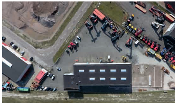
AERIAL VIEW. ON THE LEFT IS FEYTER'S CURRENT WORKSHOP AND SPARE PARTS WAREHOUSE, ON THE RIGHT THE EMPTY SPACE WHERE THE EXTENSION IS BEING BUILT.
