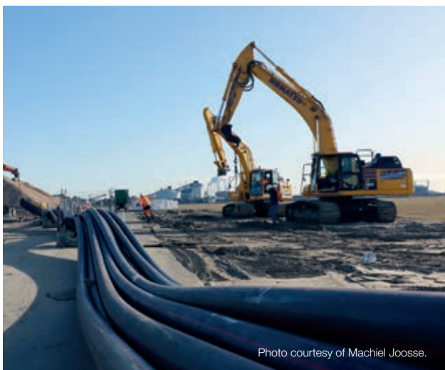
A total of two sets of twelve casing tubes were drilled. Each set has a length of 1,500m, and weighs around 350,000kg.
