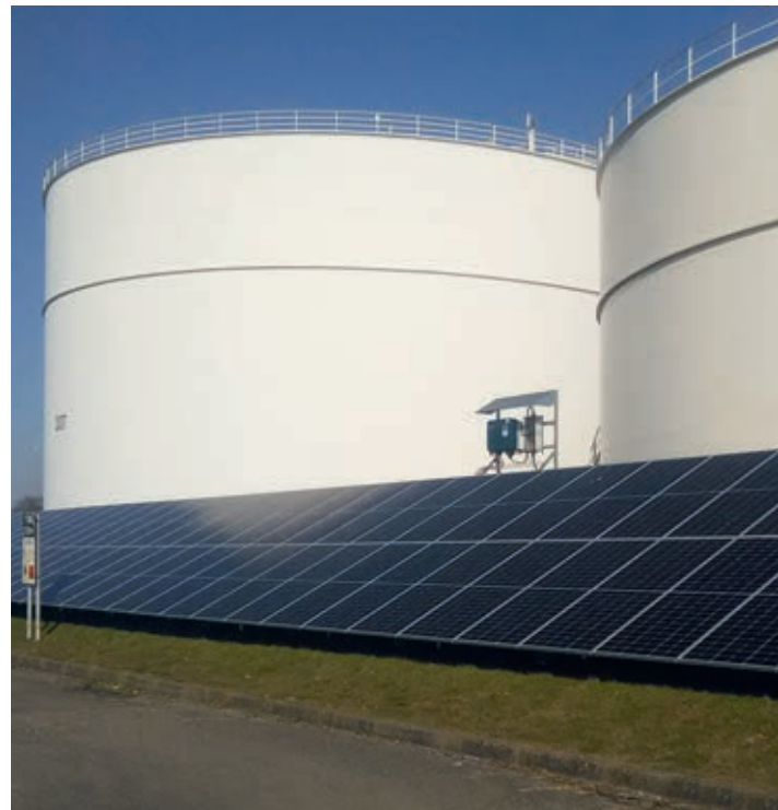
In Vlissingen, Vesta is investing in solar panels for the production of green electricity that can be used at its facilities.
