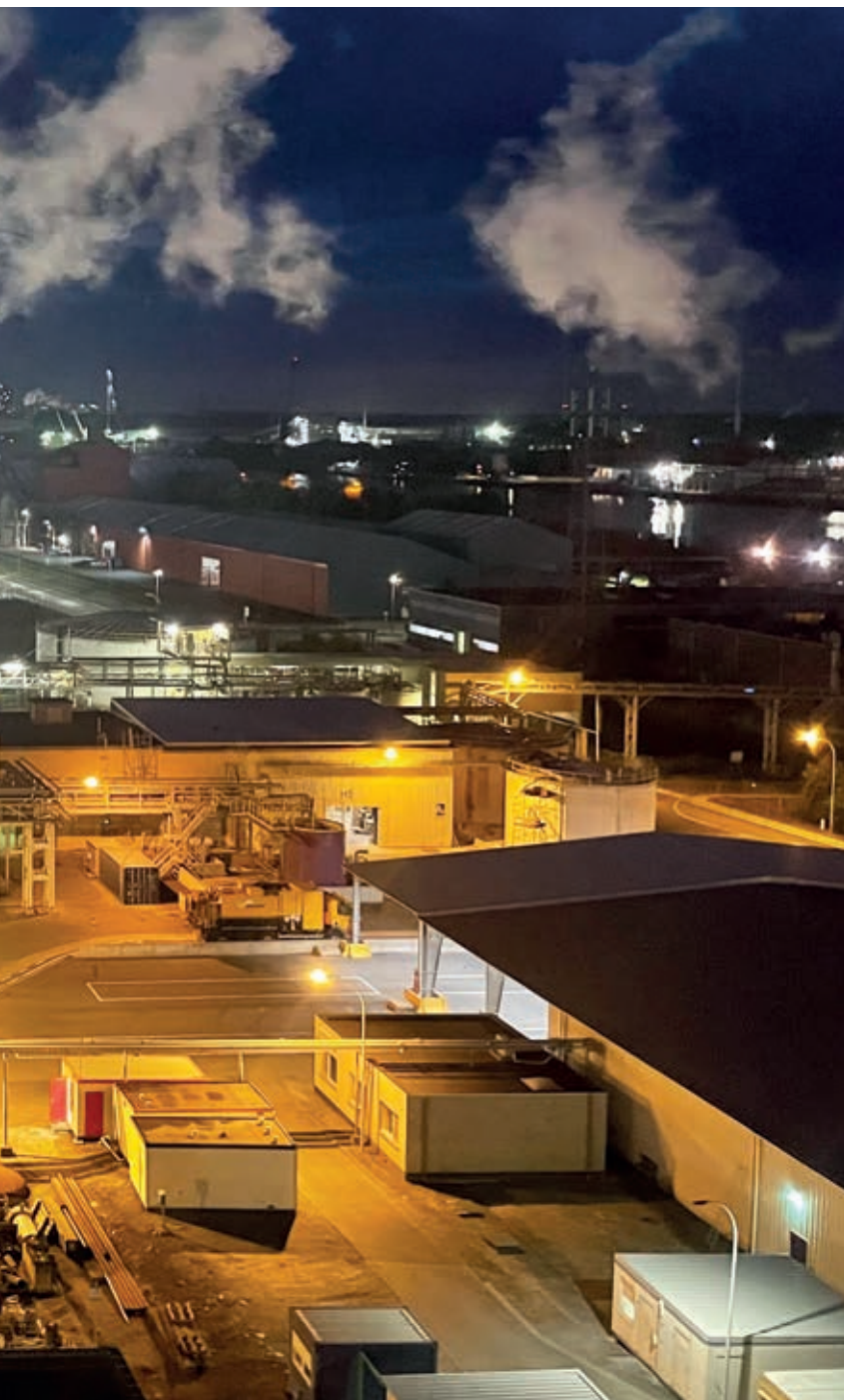
The yearly production capacity of the plant is being lifted step by step to about 120,000t.
