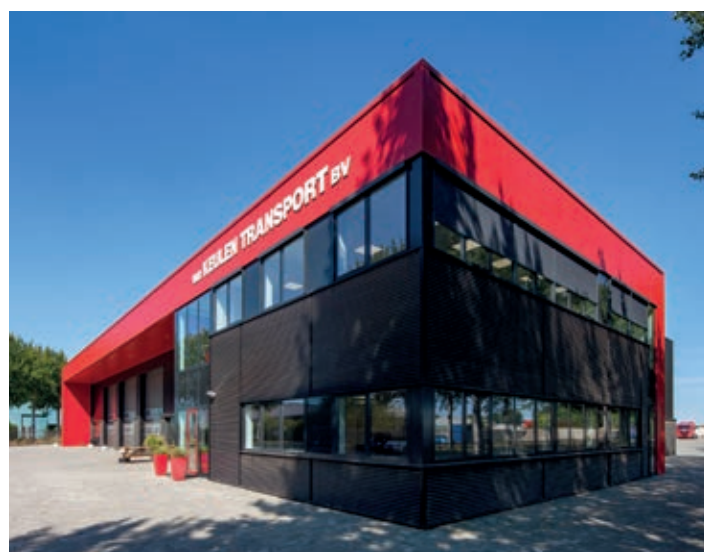
The new 1,675m 2 building for new offices and a new workshop.
