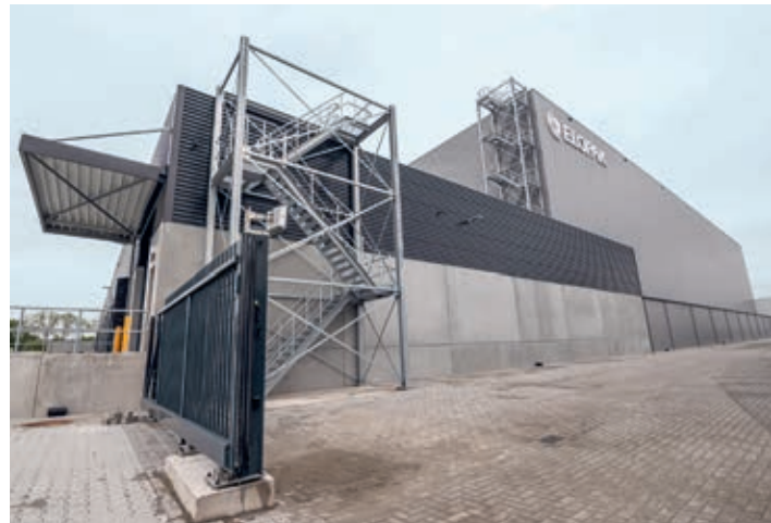
The warehouse Elopak is renting from A.C. Rijnberg Transportservice allows the company to store 480 million packages on one single location.
