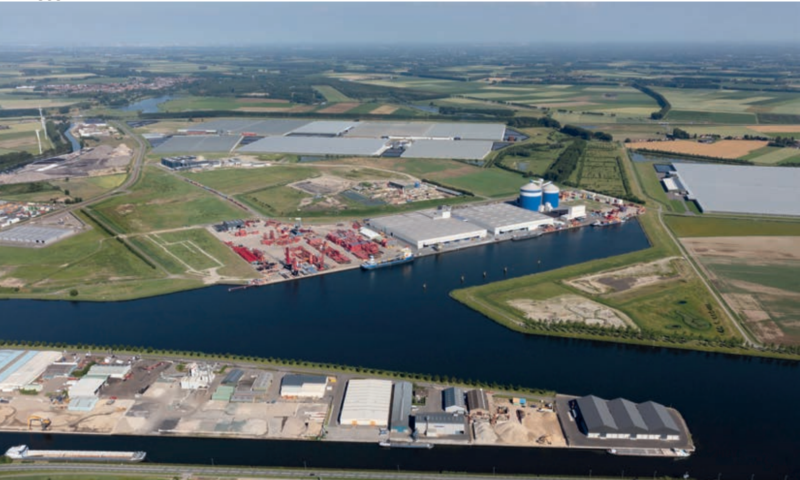
Aerial view of the Axelse Vlakte. Strategically located at the Axelse Vlakte, the project location is accessible by road, rail, and waterway to support the supply and distribution of green hydrogen to regional customers.
