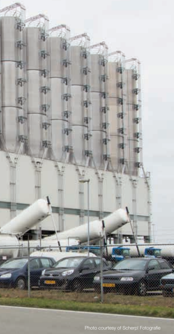
RAVAGO LOGISTICS TERNEUZEN AT VALUE PARK TERNEUZEN.
