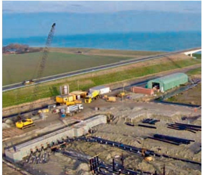
KINGFISH ZEELAND BUILDING SITE.
