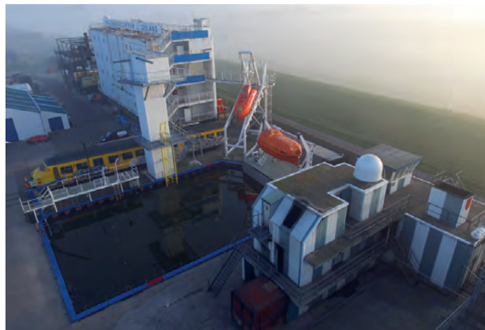
DRTC has modern and extensive training facilities to provide theoretical and practical courses.
