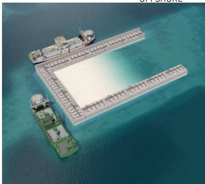
The caissons will be built and installed in 2024 and 2025 and will form the contours of the island.
