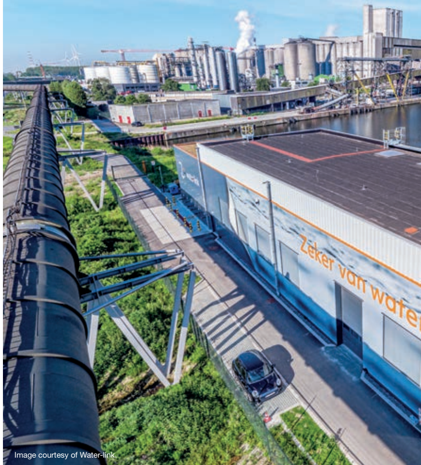
Water-link's Indus IIbis installation at the Rodenhuedok, nearby the biofuel hub where Alco Bio Fuel and Cargill have their plants
